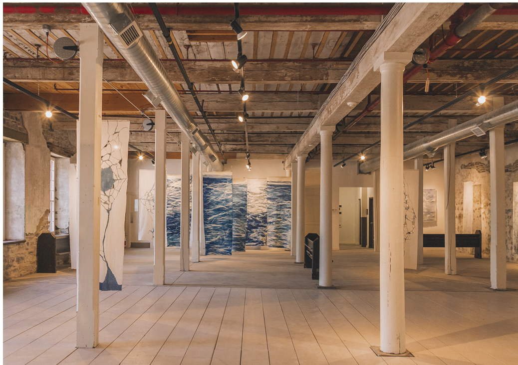
Example of Heavy Timber Construction
