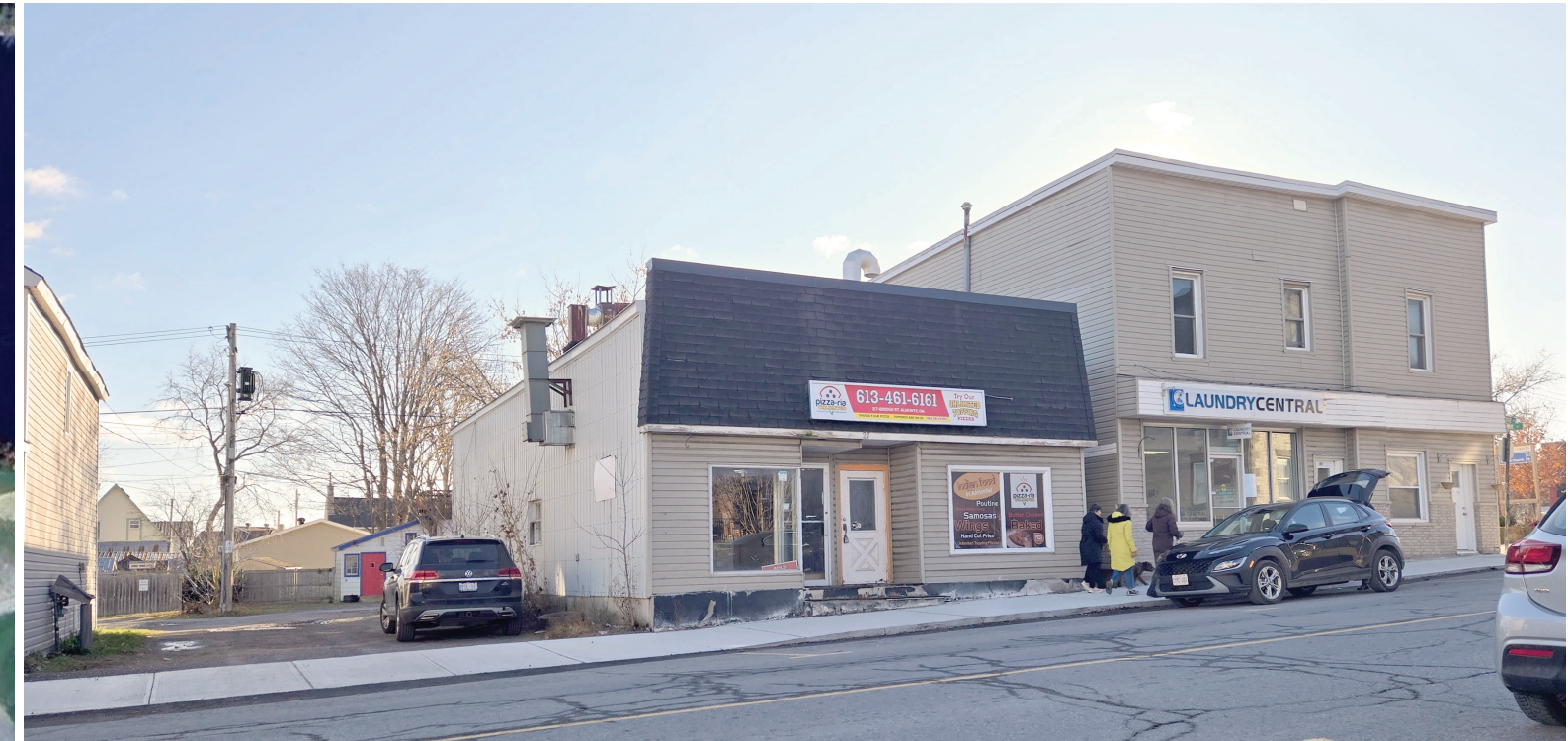
Existing Building on the Project Site
